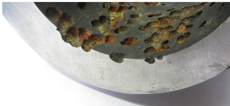
Large Corrosion Pits.
