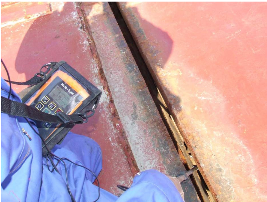
Fig 7.8. Scanning a Deep Hinged Joint.
